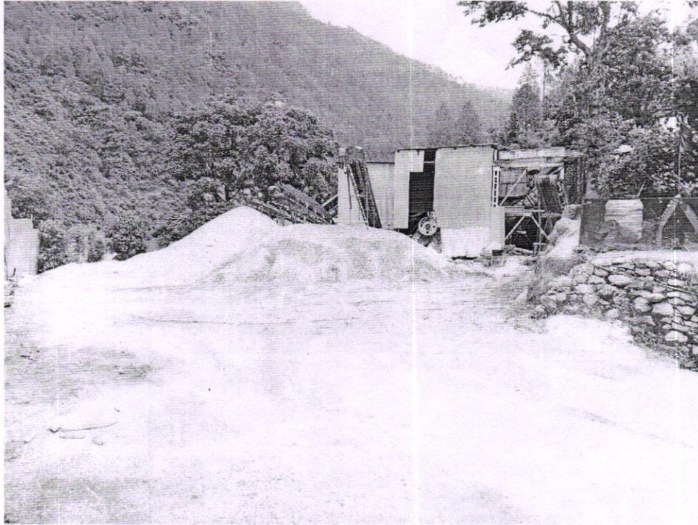
PIC 3: Stone Crusher unit
